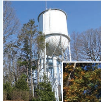
Current Water Tank at Beacon Hill.
