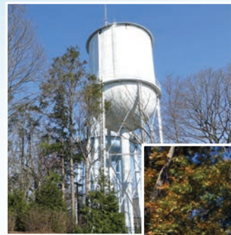
Current Water Tank at Beacon Hill.
